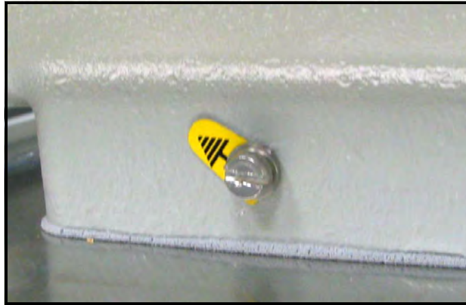
Figure 30: Earth Ground Connection
